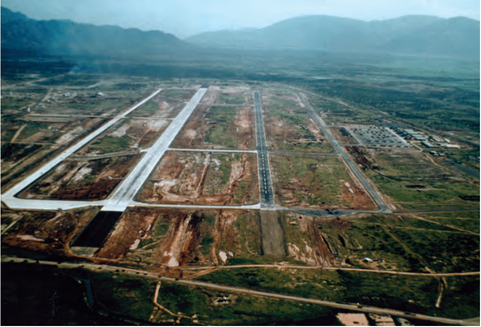
Phan Rang airfield at the end of 1966 showing concrete runway and taxiways on the left and AM2 runway on the right
